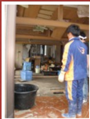
Cleaning out the mud and debris from a fisherman's house.
